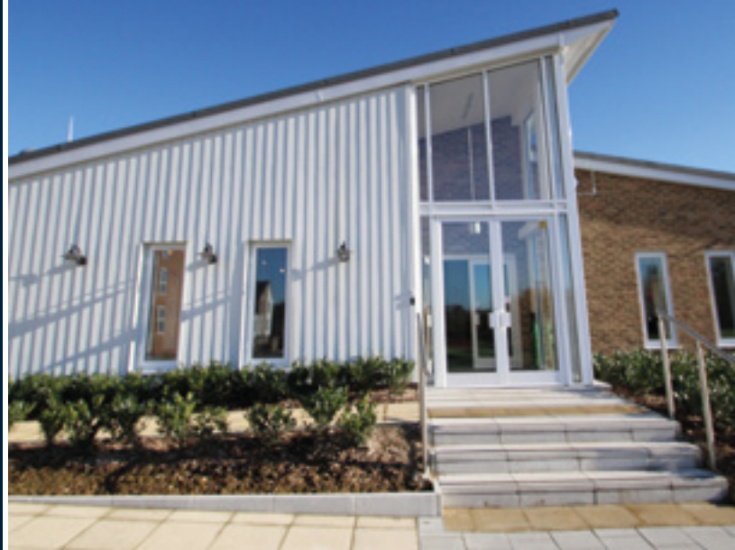
Club house, Kilnwood Vale
